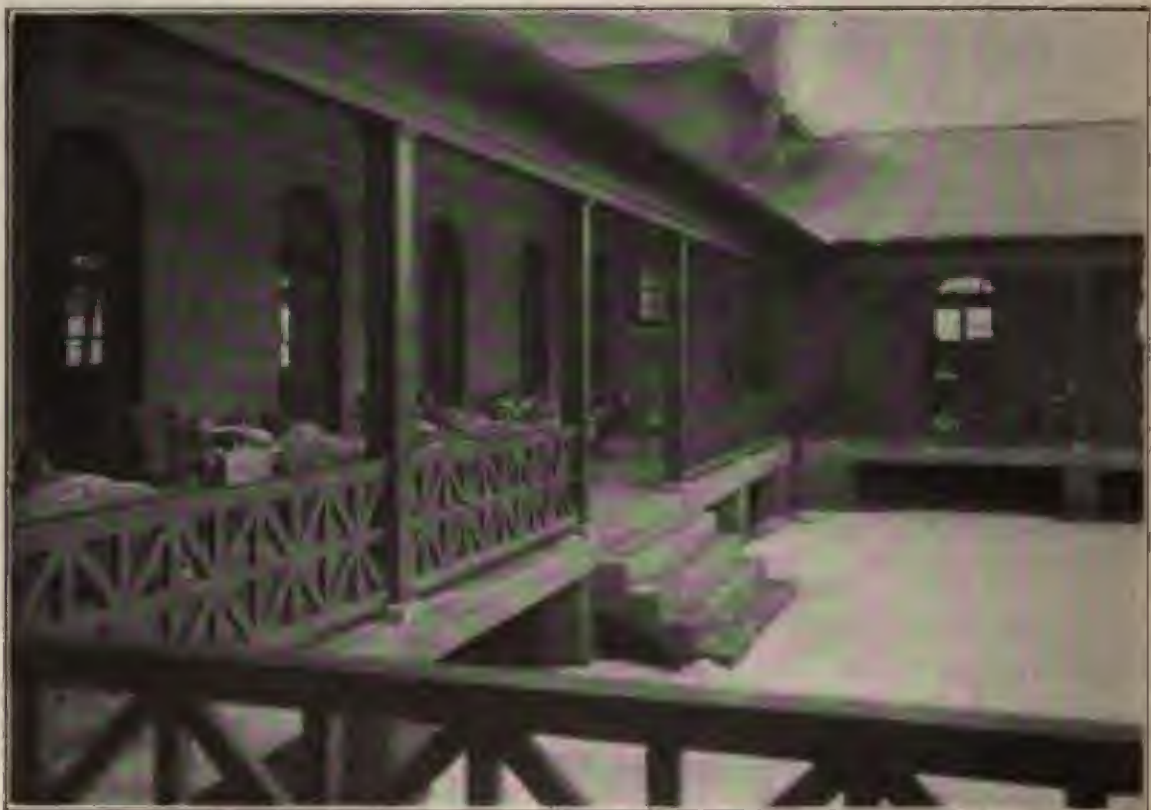
FIG. 4.—U. S. Army General Hospital, Fort Bayard, N. M. Patients sleep on the verandas in all weathers except during snow or rain storms. Note snow on roof and ground.
